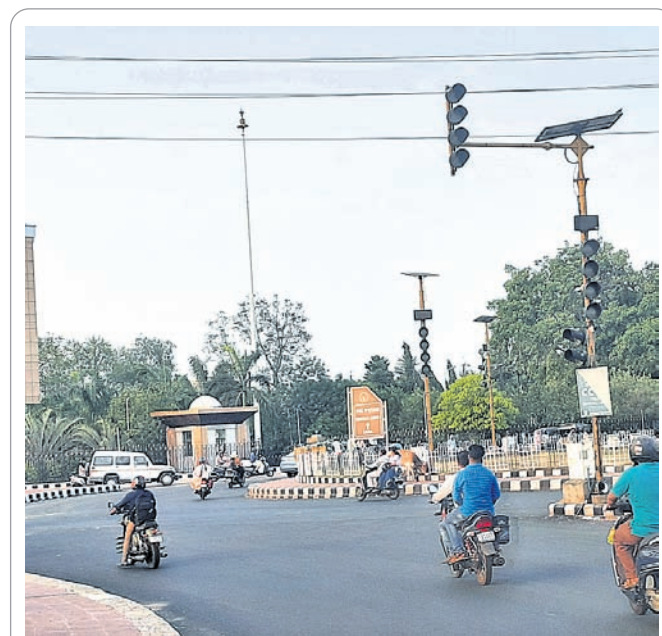
SIGNAL FAIL: A defunct traffic signal at the busy Odisha Judicial Academy intersection in Cuttack poses risk to motorists in the millennium city OP PHOTO
