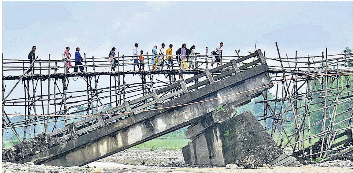
Villagers use a temporary bamboo bridge to cross a river after the RCC bridge over it washed away in flood water, at Subankhata village in Baksa district, Assam
