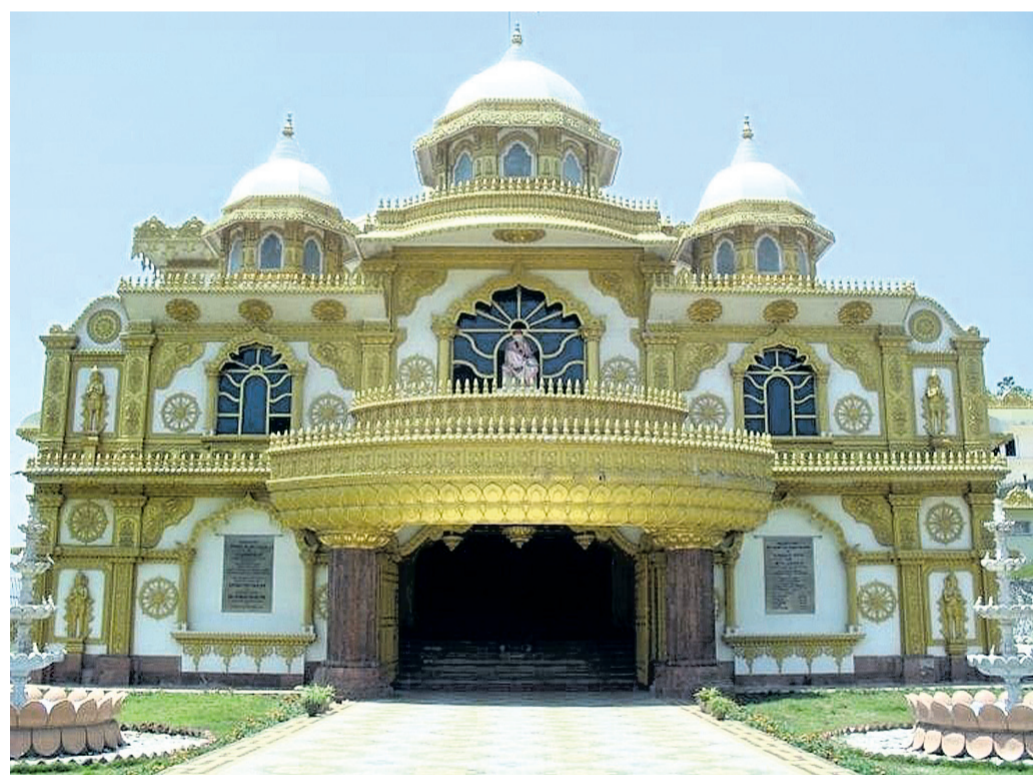
WORK OF ART: A 50-feet high puja pandal designed on the lines of Sai temple at Namchi in Sikkim put up by organisers at Block Square in Sonepur ahead of Durga Puja in this western Odisha town has been a centre of attraction
