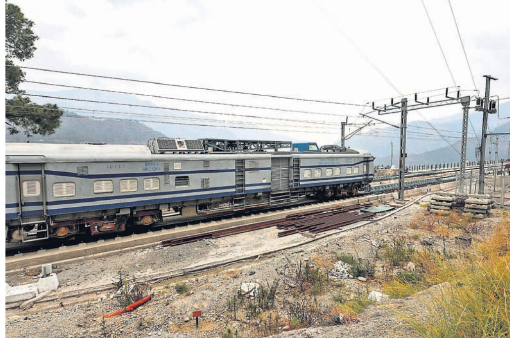
An OHE inspection car is seen on a railway track of the Chenab Rail Bridge, the world's highest railway bridge, in Reasi district, Jammu and Kashmir, Sunday, ahead of inauguration of the newly created Jammu railway division, Monday
